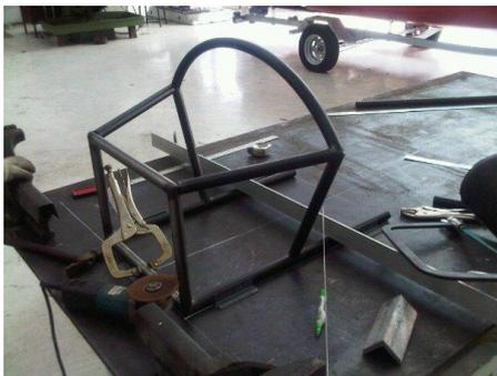
Figure 11 Section vertical welded to the frame
